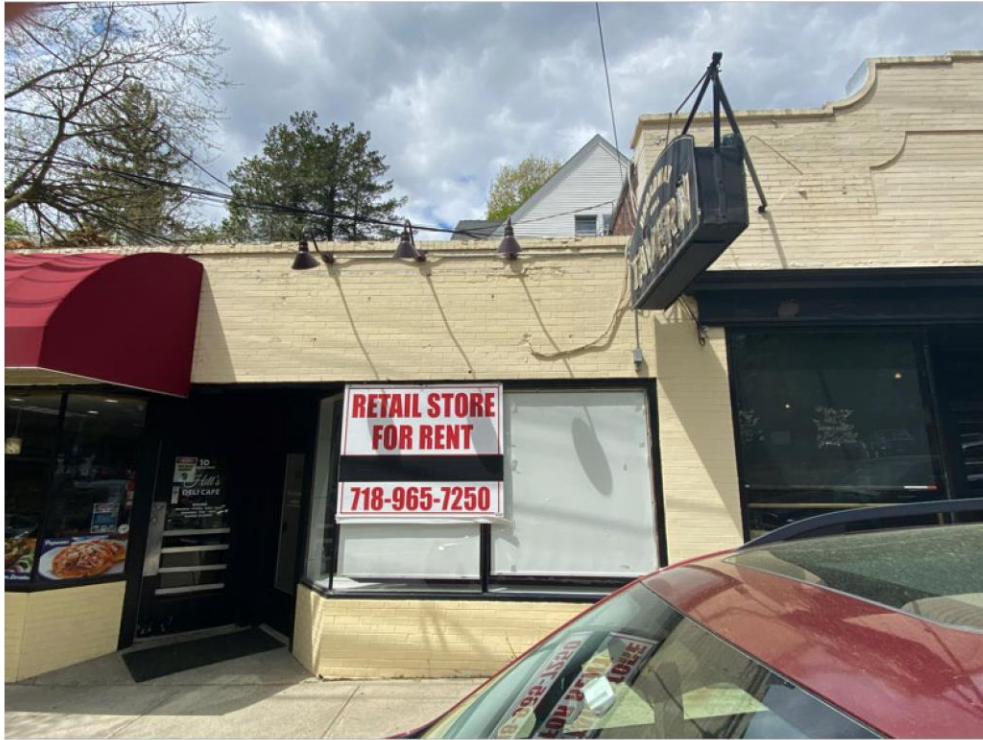
Left Adjacent Building
