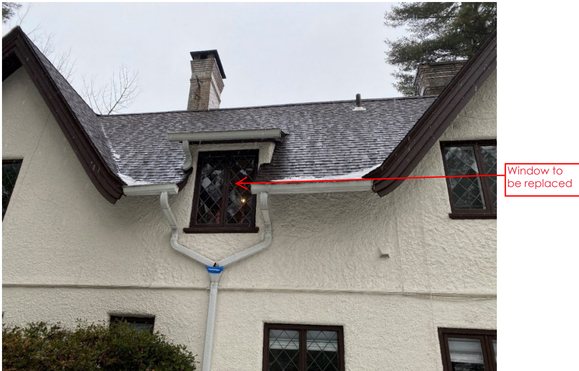
Figure 1 Image of window being replaced on Existing South Façade
