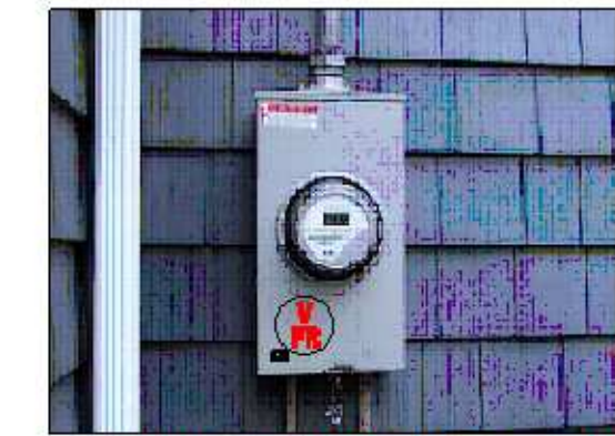
LOCATION OF FIRE ENGINEERED LUMBER WARNING SIGN SHALL BE LOCATED AS SHOWN ON ELECTRIC METER
