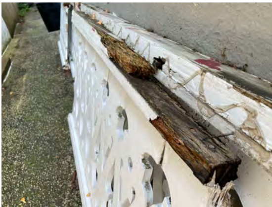
Dilapidated Railing Conditions 11
