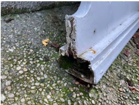
Dilapidated Railing Conditions 3
