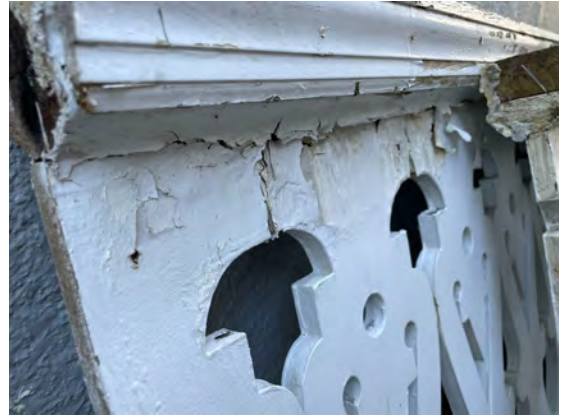
Dilapidated Railing Conditions 2
