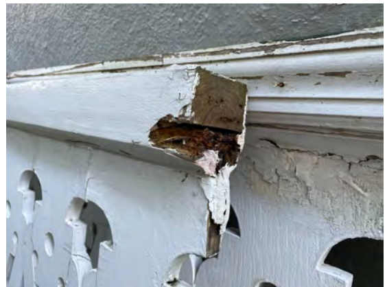
Dilapidated Railing Conditions 4
