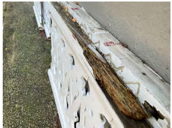
Dilapidated Railing Conditions 10
