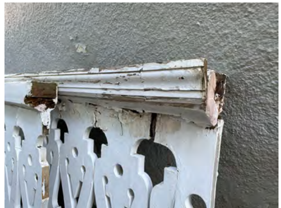
Dilapidated Railing Conditions 6
