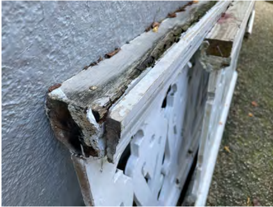
Dilapidated Railing Conditions 1
