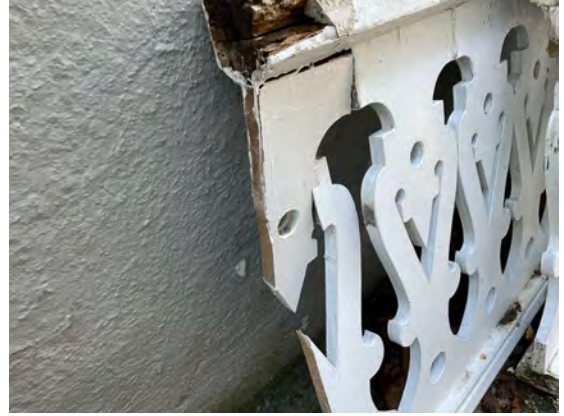
Dilapidated Railing Conditions 8
