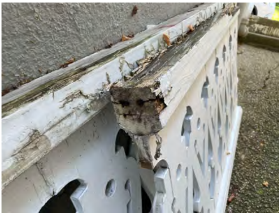
Dilapidated Railing Conditions 9
