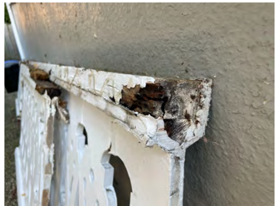
Dilapidated Railing Conditions 12
