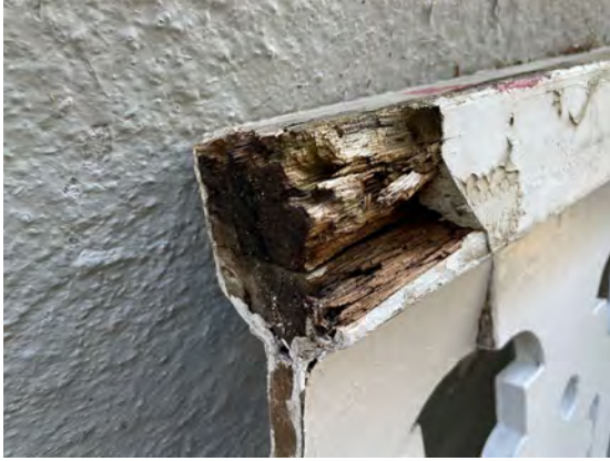
Dilapidated Railing Conditions 7
